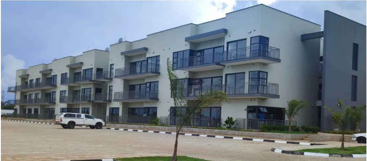
Millennium Heights Block 2 - Completed & Handed Over in December 2022
