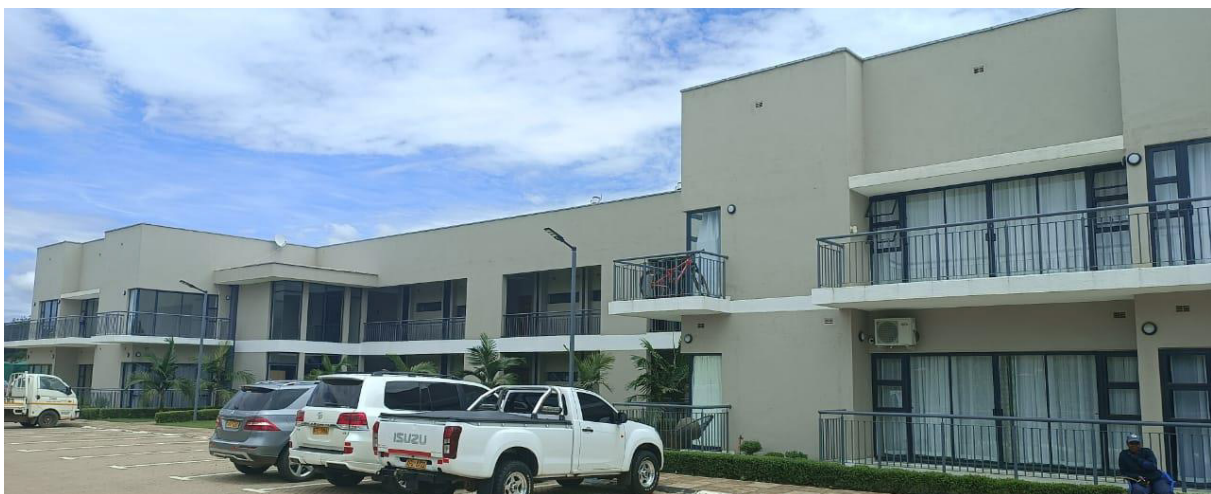
Millennium Heights Block 1 - Completed & Handed Over in June 2021
