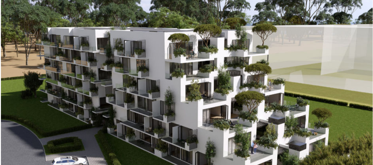
Millennium Heights Block 4 – Pipeline
