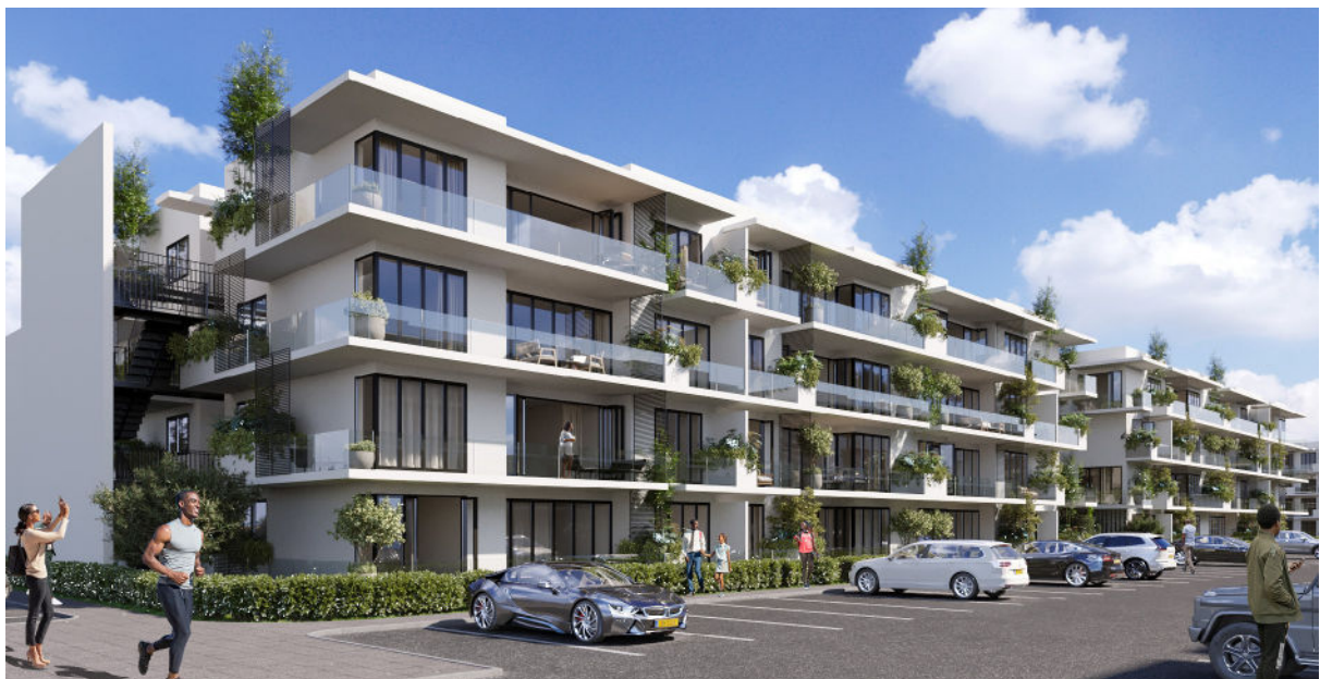
Millennium Heights Block 3 - Under Development
